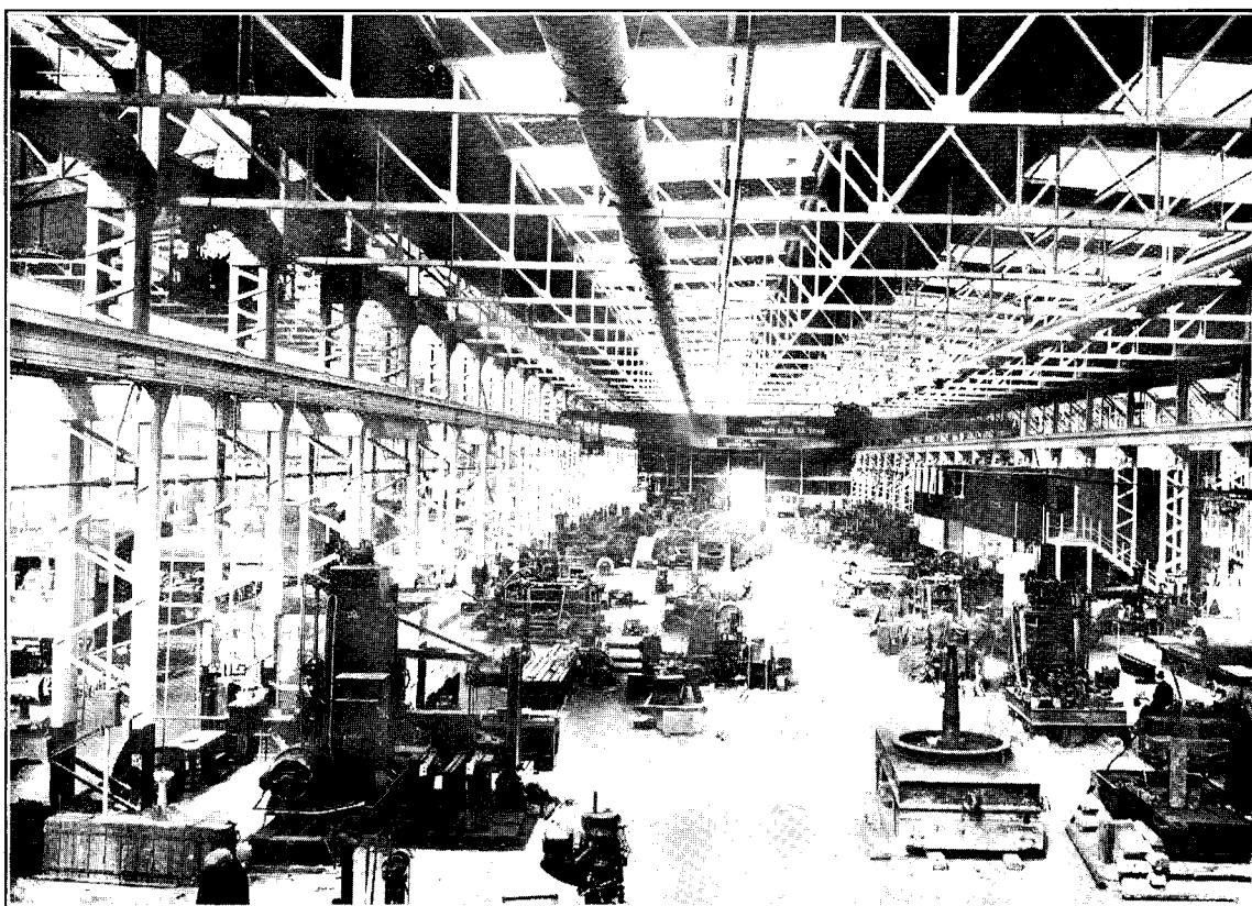
HEAVY-MACHINE SHOP, HUTT VALLEY.
