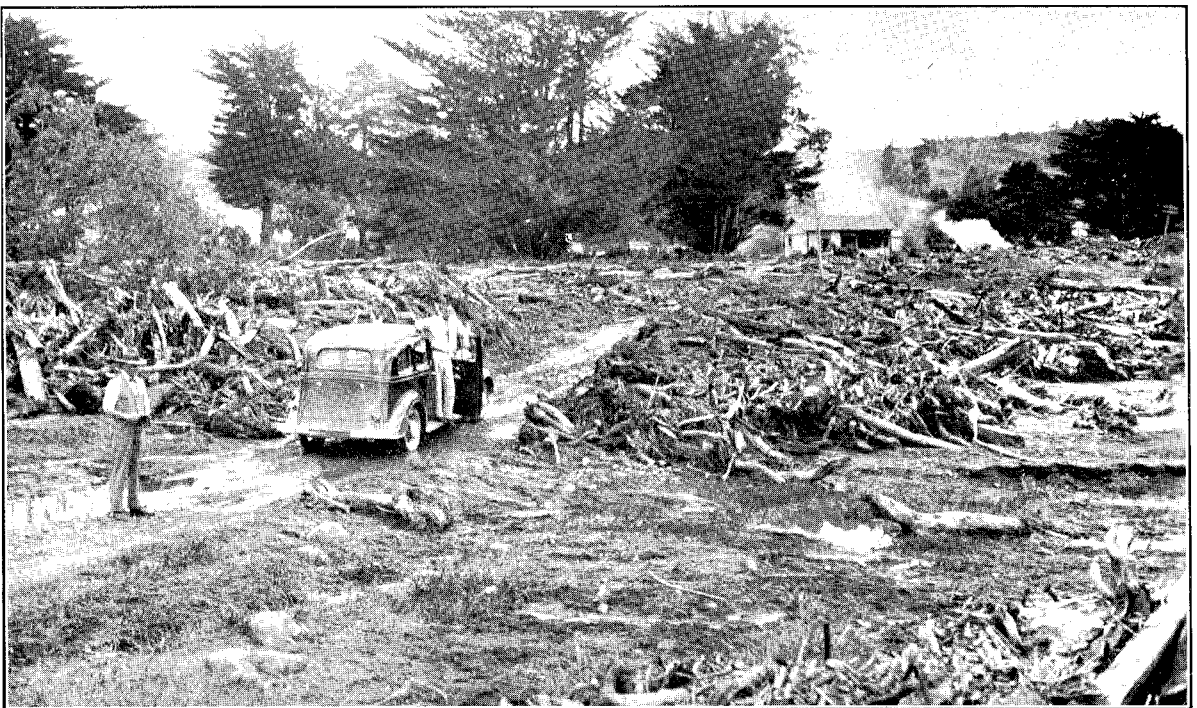
SCENE AFTER FLOOD. WAIMAMAKU—OHAEAWAI MAIN HIGHWAY.
