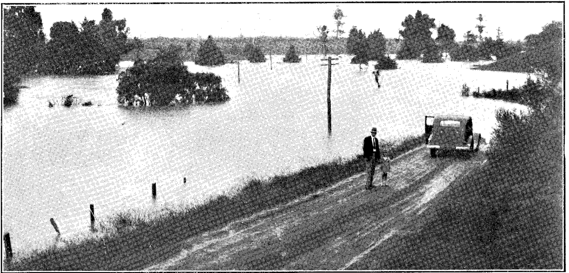
SAME SECTION UNDER FLOOD. WAIPAPAKAURI—MAUNGATAPERE MAIN HIGHWAY.
