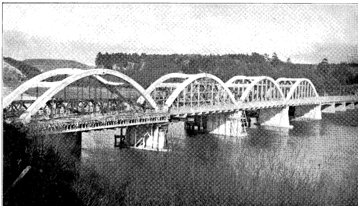
FITZHERBERT BRIDGE OVER MANAWATU RIVER. LEVIN—PALMERSTON NORTH, VIA SHANNON, MAIN HIGHWAY.
