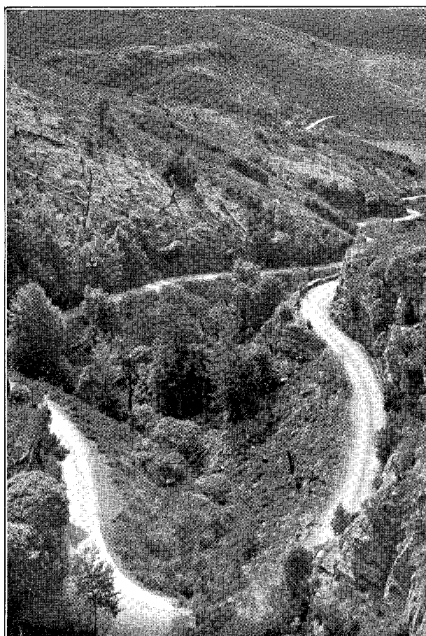
BAD BEND TO BE ELIMINATED BY DEVIATION.—TAKAKA HILL, HAWKE'S CRAIG SECTION. RICHMOND—COLLINGWOOD MAIN HIGHWAY.
