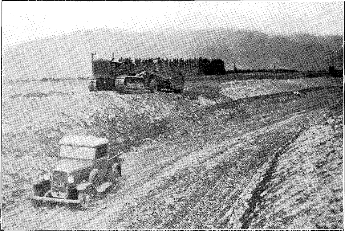
RANGITATA DIVERSION RACE. BANKS BEING BUILT BY TRACTOR-DRAWN CARRY-ALL SCRAPER.
