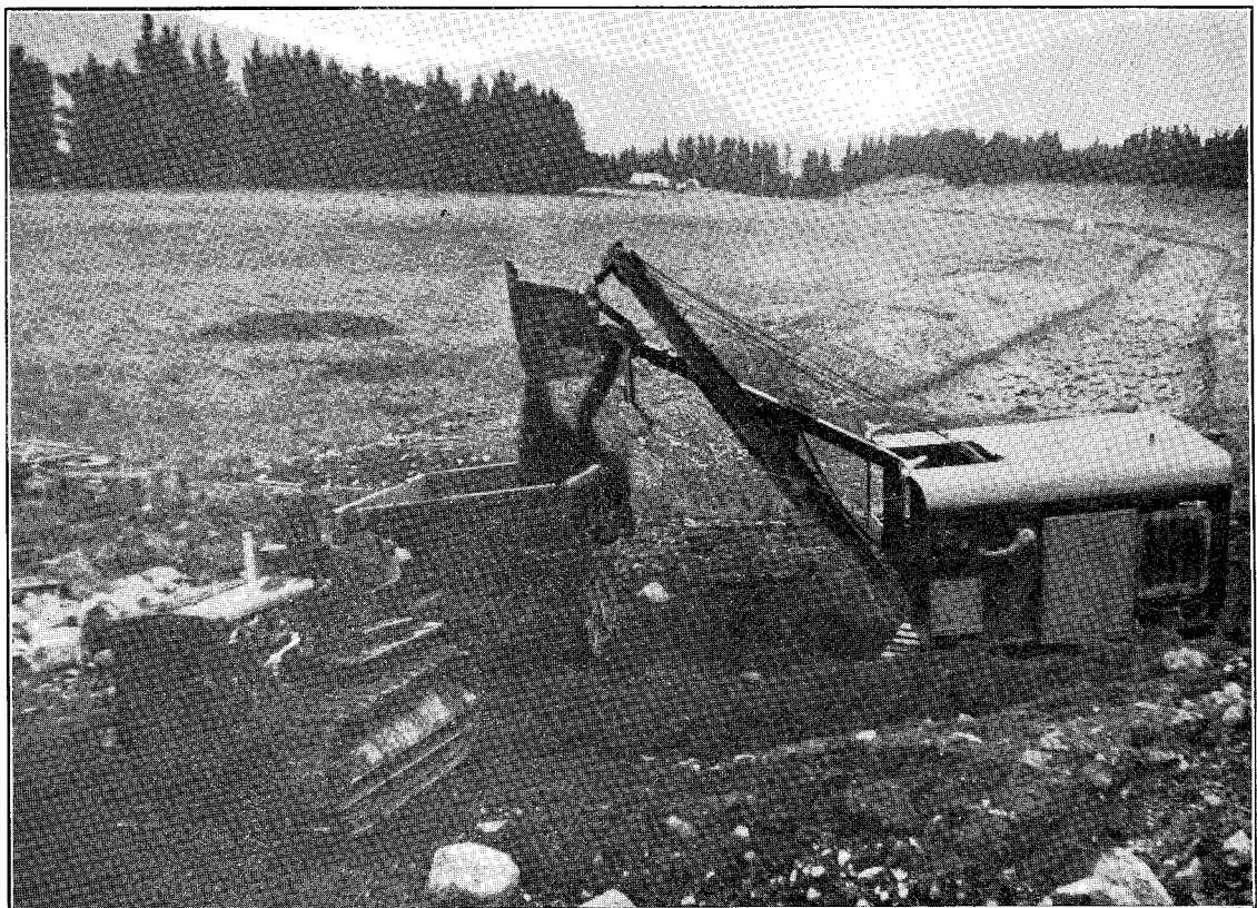
RANGITATA DIVERSION RACE. HIGH-SPEED SHOVEL LOADING 10-CUB.-YD. TRUCK. ASHBURTON-LYNDHURST IRRIGATION SCHEME.
