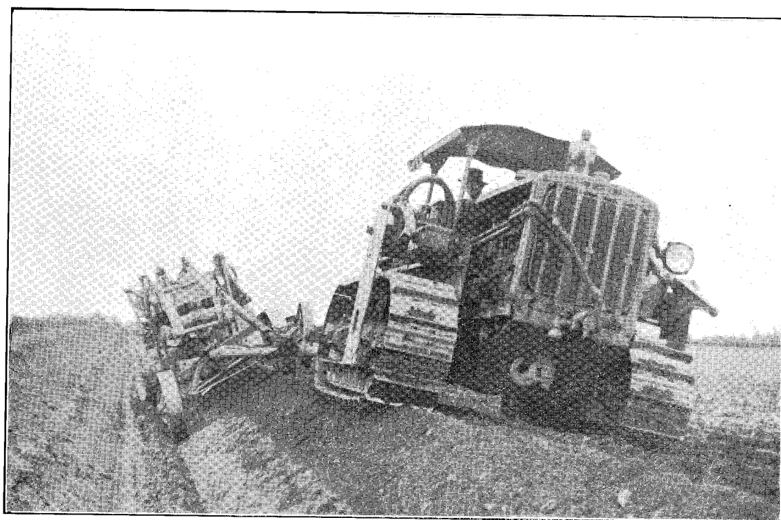
TRACTOR AND GRADER FORMING DISTRIBUTARY RACE. ASHBURTON-LYNDHURST IRRIGATION SCHEME.
