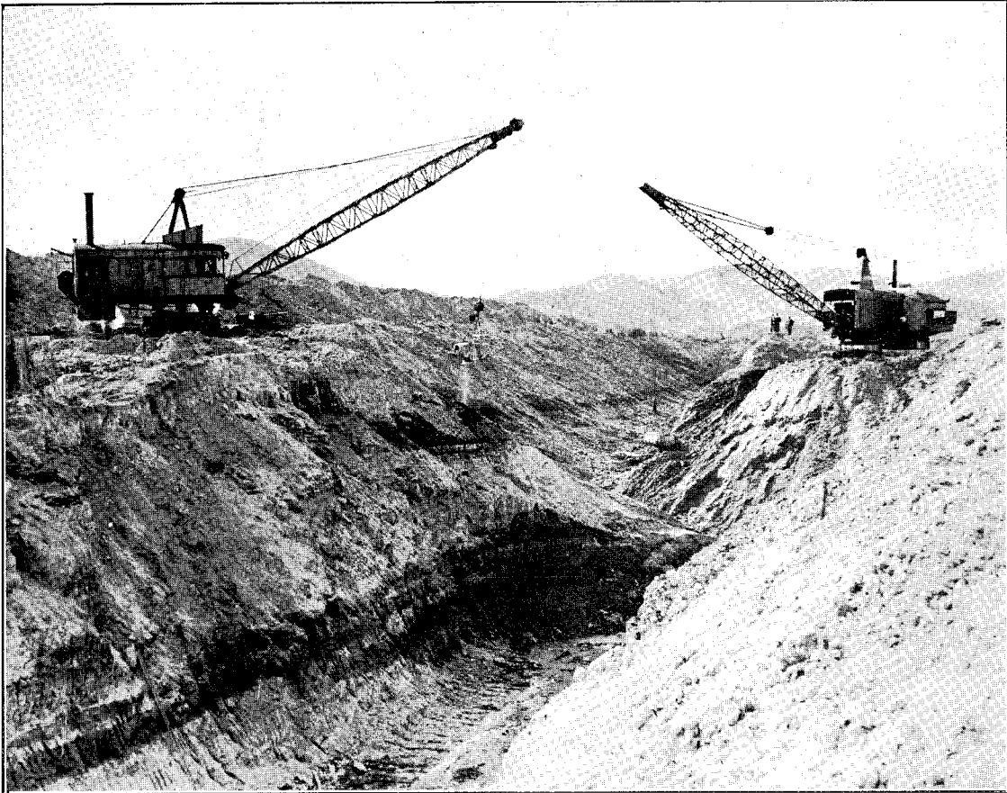
DRAG-LINE EXCAVATORS, 1\frac{1}{2} -CUB.-YD. CAPACITY, IN OPERATION, HAWKESWOOD CUTTING.
