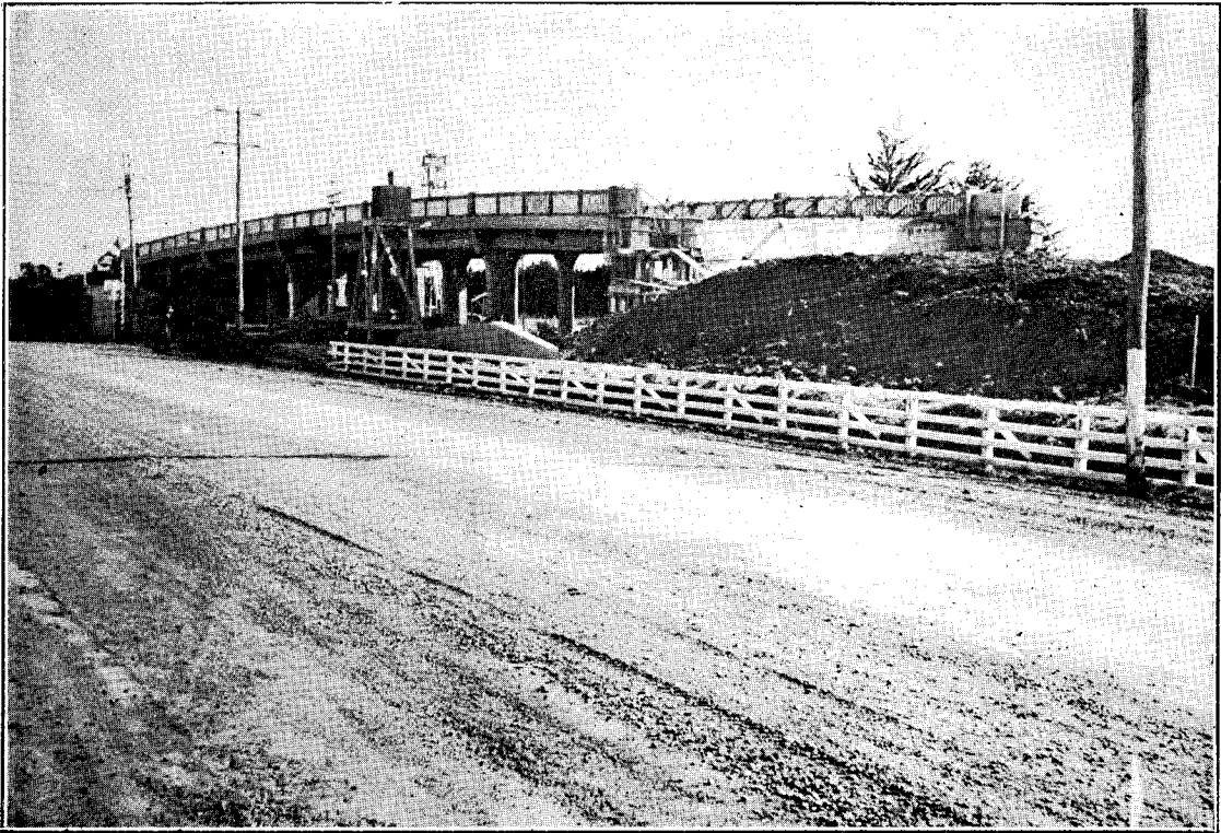
LORNEVILLE OVERBRIDGE, WHICH WILL ELIMINATE A HEAVILY-TRAFFICKED LEVEL-CROSSING.
