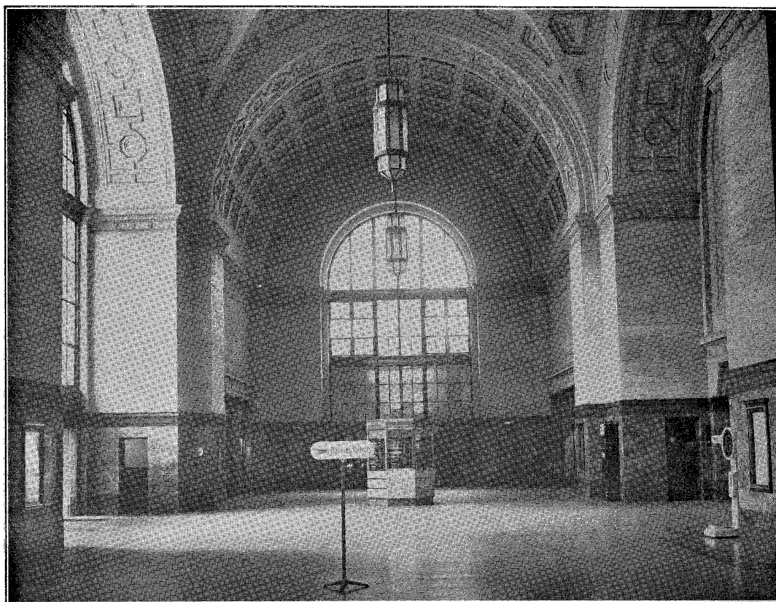
MAIN BOOKING-HALL, WELLINGTON NEW STATION.
