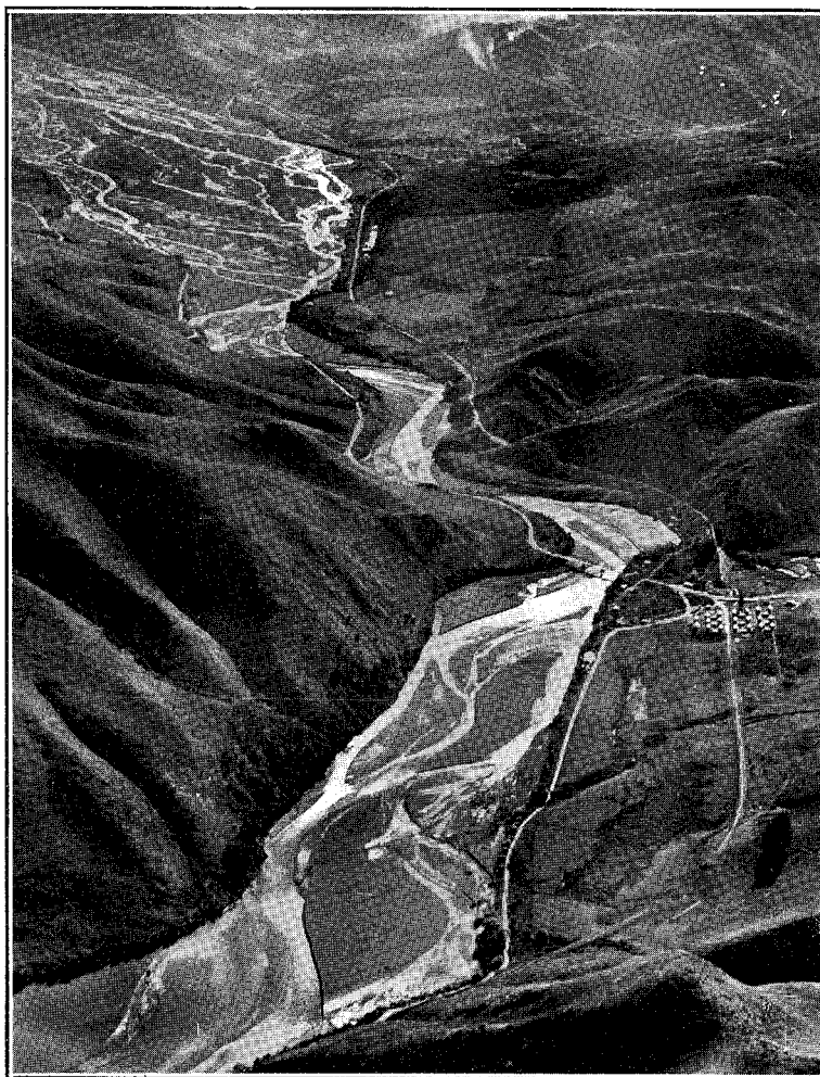
AERIAL VIEW LOOKING UP CONWAY RIVER, SHOWING RAILWAY-FORMATION AND ROAD. P.W.D. CAMP ON RIGHT.
