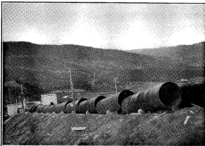
6 FT.-DIAMETER STEEL PIPES READY FOR LINING-UP AND WELDING.
