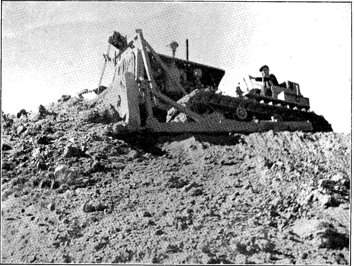
“ ANGLE-DOZER ” OPERATING ON ROAD-FORMATION.
