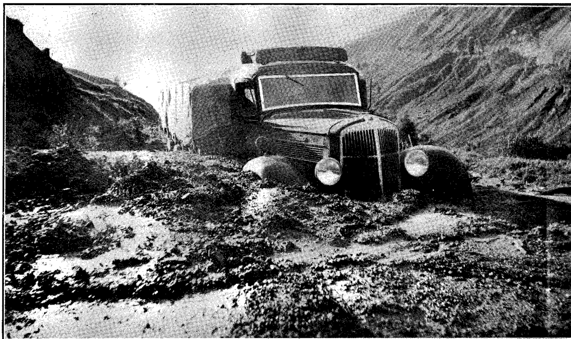
MAIL-CAR TO NAPIER CAUGHT IN LARGE SLIP DURING FLOODS, MAY, 1938.
