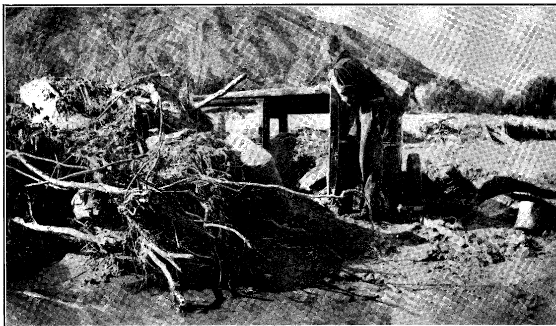
TYPICAL SILTATION DURING FLOODS, MAY, 1938. GISBORNE-NAPIER VIA HANGAROA STATE HIGHWAY.
