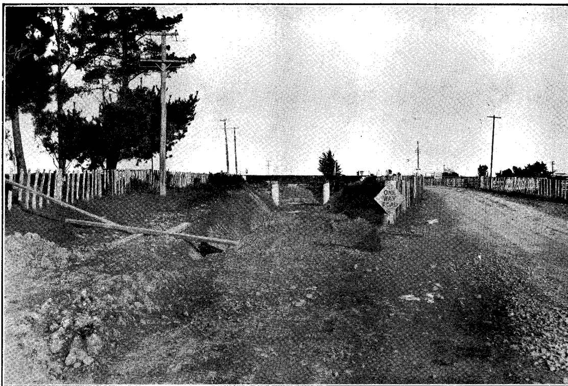
CLIFF ROAD SUBWAY. VIEW LOOKING SOUTH SHOWING TEMPORARY ROAD ON RIGHT. HOROPITO-BULLS VIA TAIHAPE STATE HIGHWAY.
