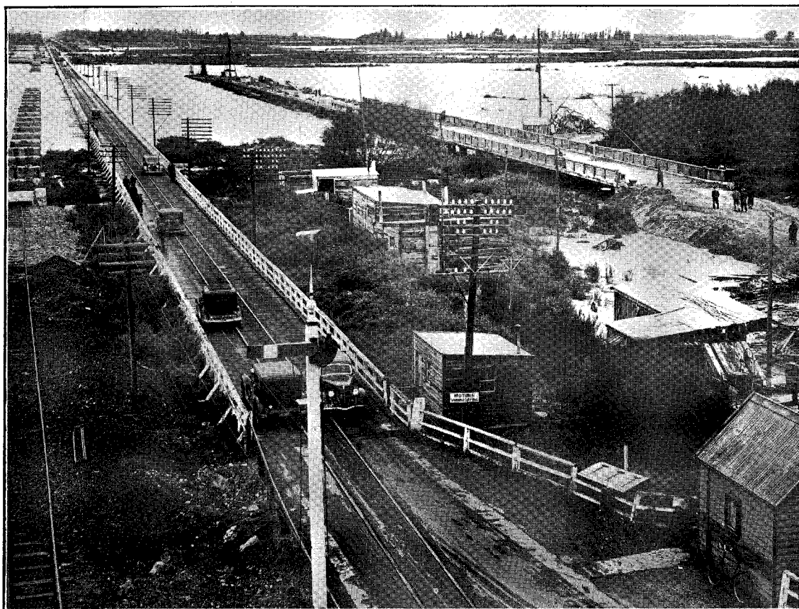
RAKAI RIVER ROAD BRIDGE, 5,760 FT. IN LENGTH, 24 FT. ROADWAY, UNDER CONSTRUCTION ON RIGHT. NOTE NEW RAILWAY-BRIDGE UNDER CONSTRUCTION ON EXTREME LEFT AND EXISTING COMBINED ROAD AND RAILWAY BRIDGE IN CENTRE.
