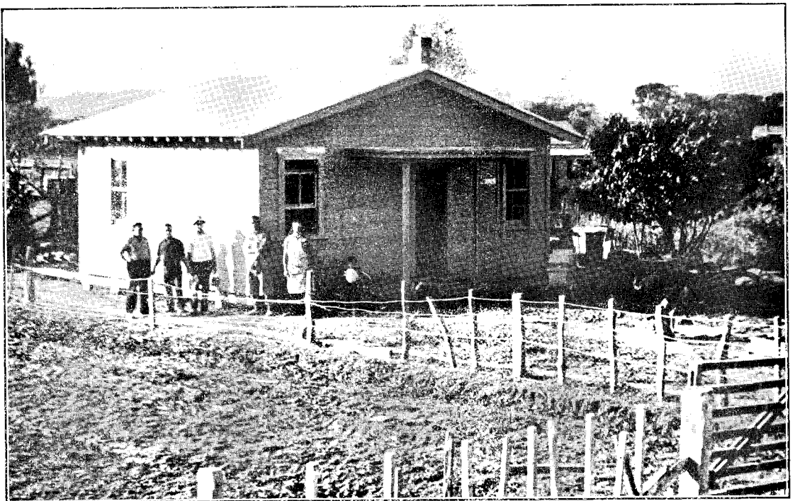
26. HOUSING SCHEME: NEW COTTAGE NEARING COMPLETION, BUILT ON THE SAME SETTLER'S SECTION.
