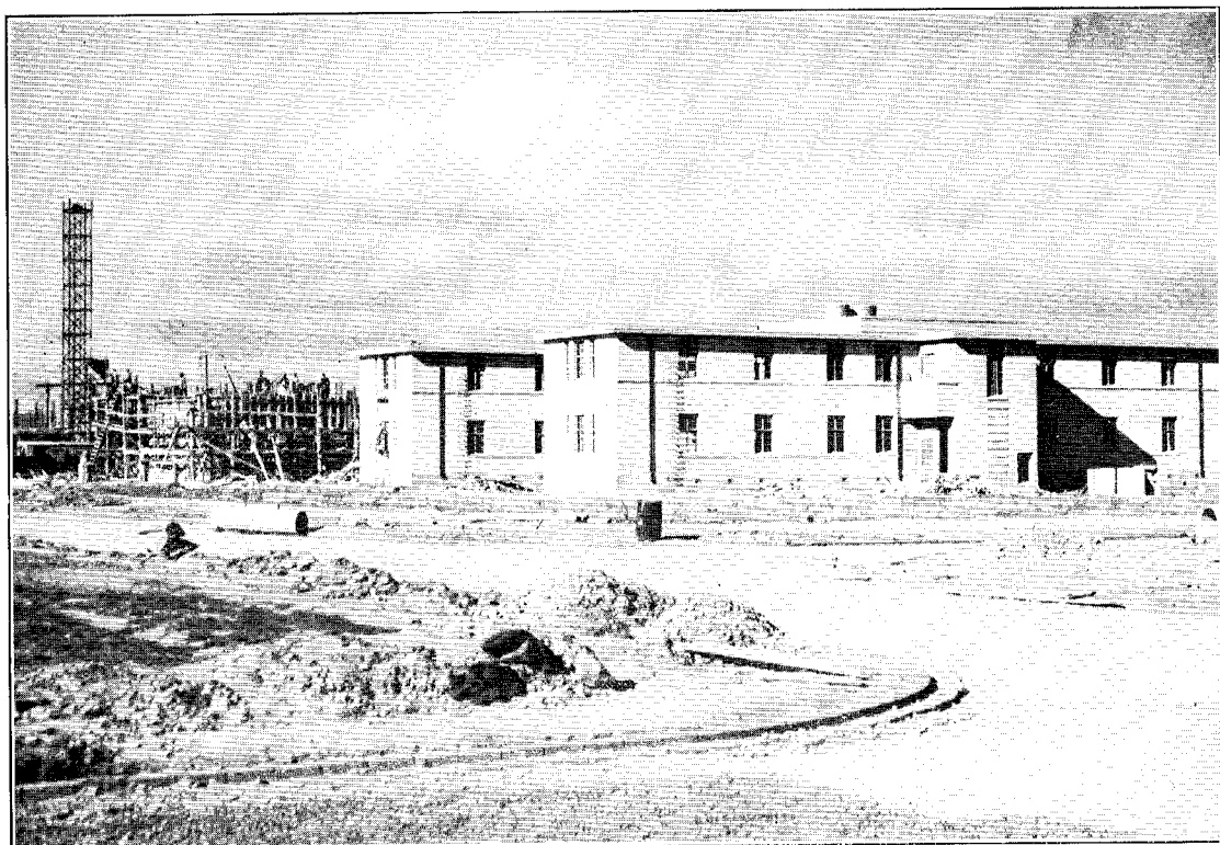
R.N.Z.A.F. STATION, OHAKEA : AIRMEN'S BARRACKS UNDER CONSTRUCTION.
